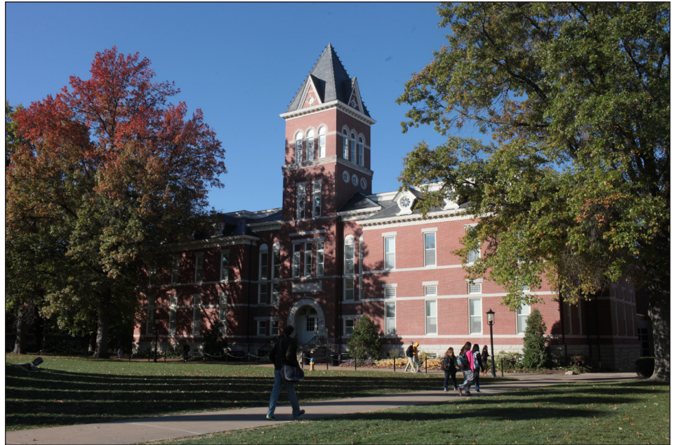
Thomas and Nell Lafferre Hall is currently undergoing a major renovation that is slated to be completed in December 2016.
